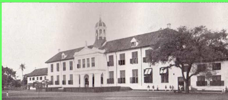
P. 4. Town Hall in 1911, two dormer-windows
